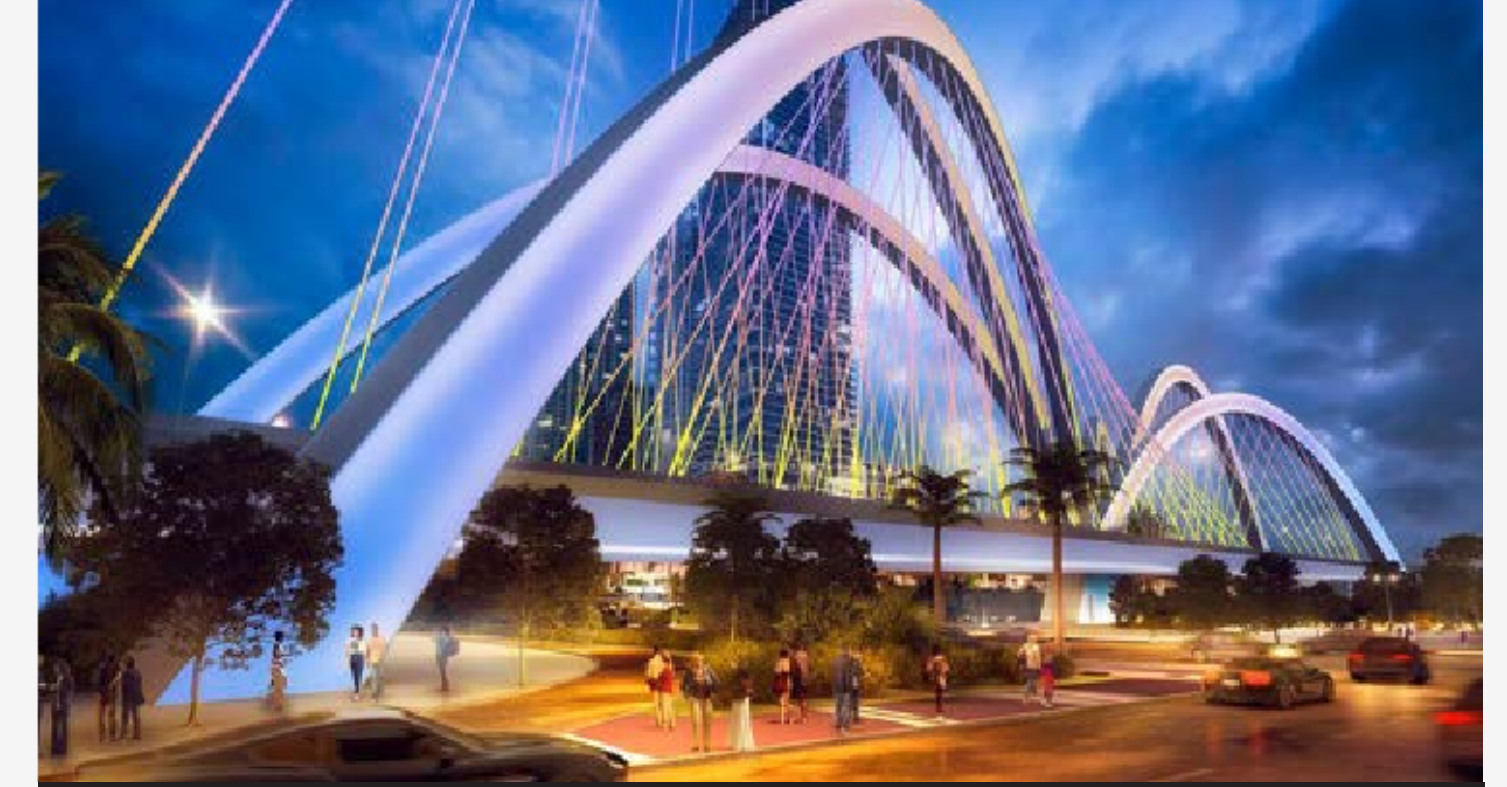
I-395 Signature Bridge
